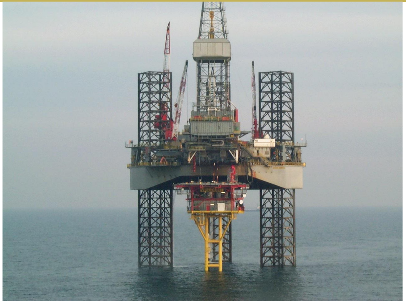
Letourneau 116C class drilling rig over a Southern North Sea Normally Unmanned Installation.
