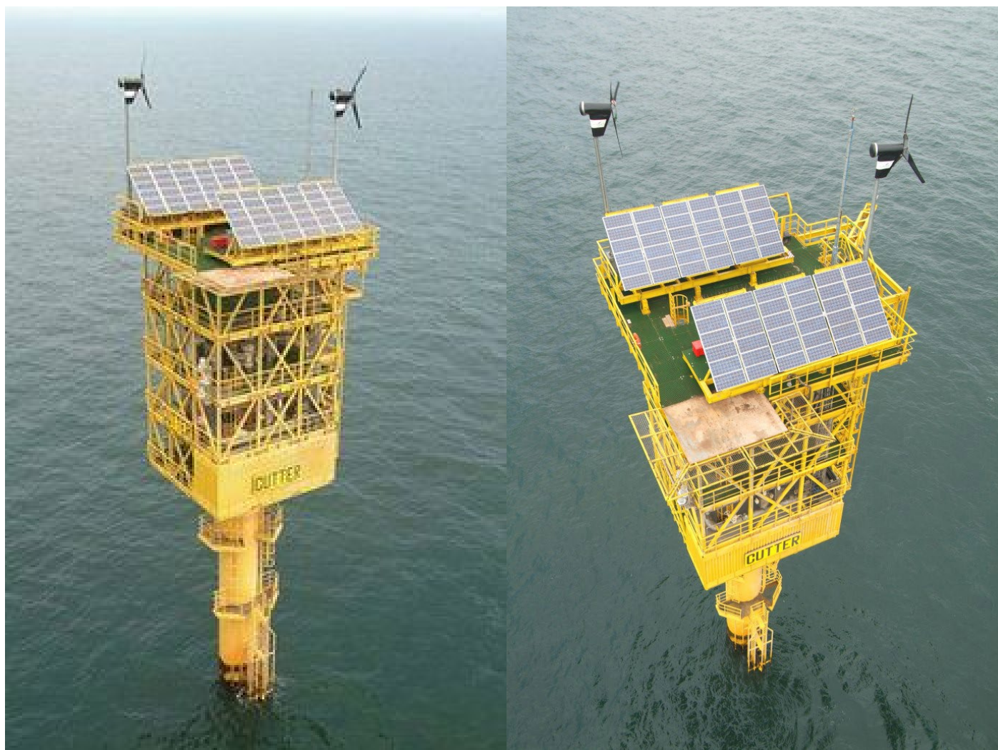
Figure 11 - Example Monopod Jacket usable with Dry Surface Trees
