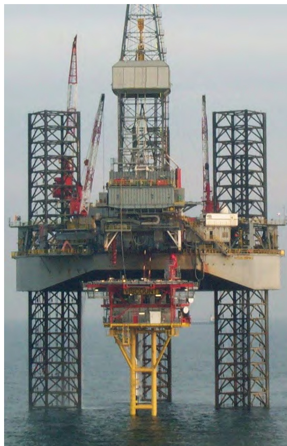
Figure 2 - LeTourneau 116C Class Drilling Rig over a Small Platform in UK Southern North Sea
