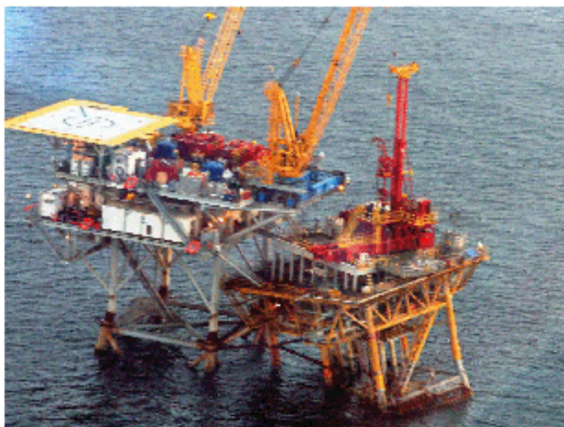
Figure 10 - Rigless Pulling & Jacking Unit (PJU) on damaged platform well (Canny, 2017) 17
