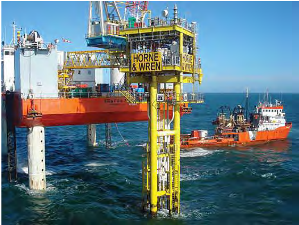
Figure 4 - Barge Bridge Linked to UK SNS Horne Wren Platform (Tullow) 48
