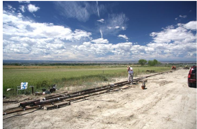
Figure 2 – Boneyard Test Facility
